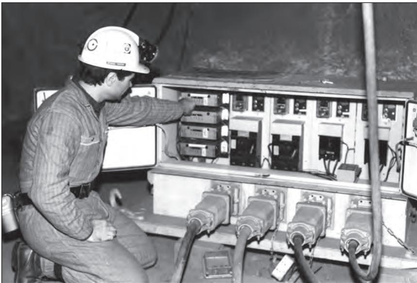
**Figure 6. Sensitive AC GFR's installed in Safety Research Coal Mine**
