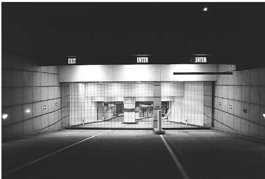
Figure 5.8 An open-grille roll-down gate leading to a subterranean parking garage. Photograph by Stephen Lo.
