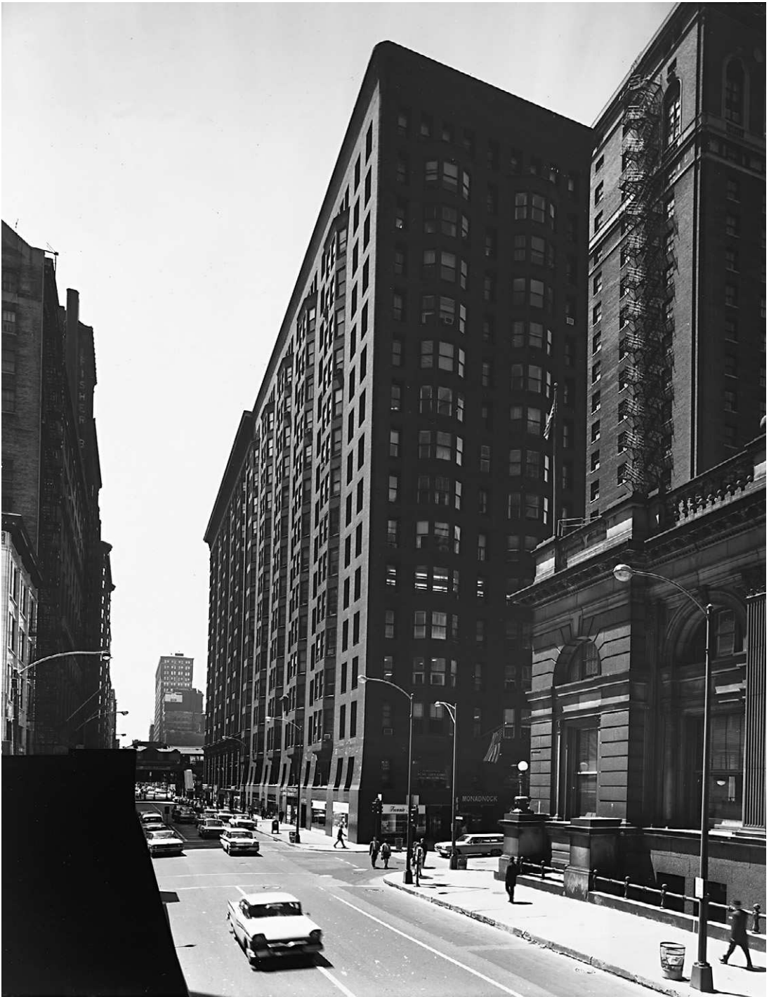
Figure 1.1 Monadnock building. This 16-story building is the tallest load-bearing brick structure in the world. At their base, the building walls are 6 feet thick. Courtesy of the Chicago Historical Society.
