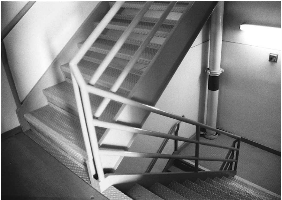
Figure 5.9 Interior of a typical emergency exit stairwell in a modern high-rise building. Photograph by Stephen Lo.
