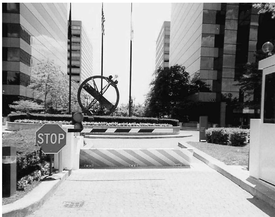
Figure 5.5 A fully raised 2-foot high crash-rated, surface-mounted steel barricade is “capable of taking axle loadings in excess of any permitted North American or European road transport vehicles” (Delta Scientific Corporation). Courtesy of Delta Scientific Corporation.
