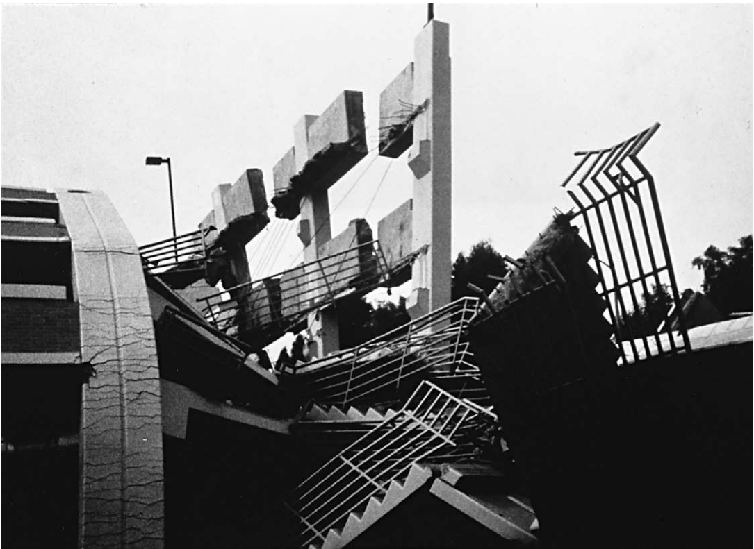
Figure 10.16 TOTAL DESTRUCTION. Severe shaking during the 1994 Northridge earthquake led to the collapse of this recently constructed, precast four-level concrete parking structure at California State University. Courtesy of Los Angeles Fire Department, Disaster Preparedness Division.
