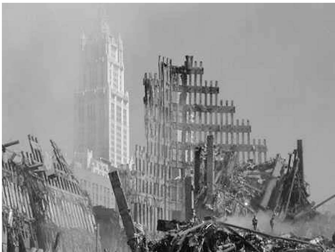
Figure 10.14 UTTER DEVASTATION. The Woolworth Building rises behind the rubble of the collapsed World Trade Center buildings in New York on September 18, 2001. Used with permission from FEMA News Photo (Photograph by Michael Rieger).
