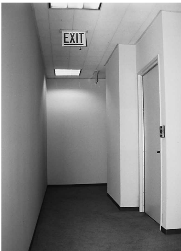
Figure 11.18 Exit sign indicates the stairwell entrance.
