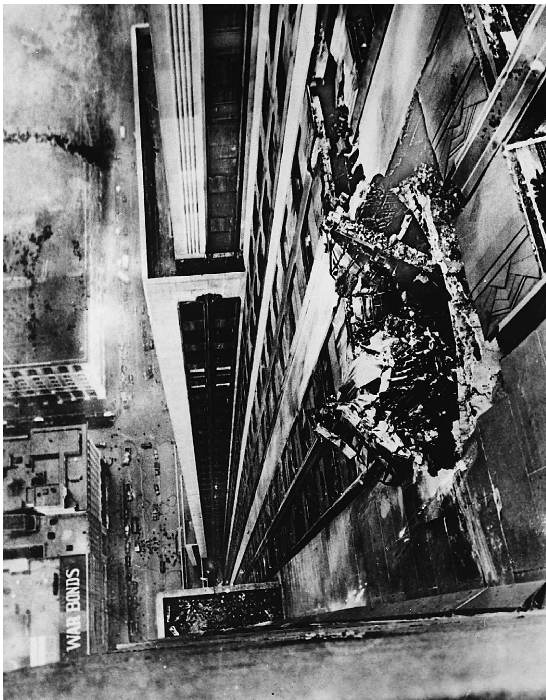
Figure 10.10 BOMBER STRIKES THE EMPIRE STATE BUILDING—A view from an upper floor of the building vividly shows the gaping hole at the 79th floor created by the impact of a B-25 bomber. Part of the wreckage of the plane, which crashed into the building on July 28, 1945, protrudes from the opening. Used with permission from AP/WIDE WORLD PHOTOS.
