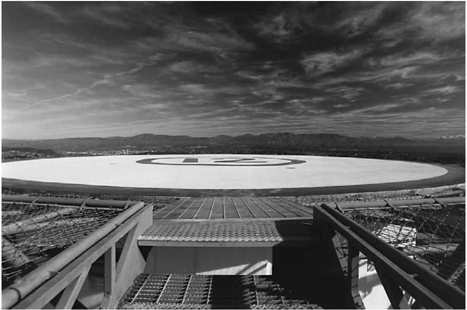
Figure 11.4 Helipad of a modern high-rise building. Photograph by Roger Flores.
