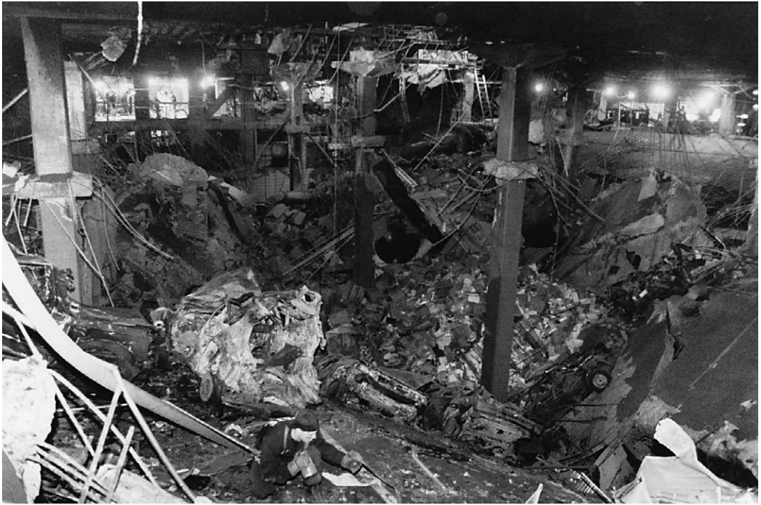
Figure 10.5 DEVASTATION AT THE WORLD TRADE CENTER. Patient sifting through the debris of the severely damaged subterranean parking garage of the World Trade Center led investigators to the discovery of a vehicle identification number from the van that contained the explosives used in this horrific bombing on February 26, 1993. Courtesy of the Department of the Treasury, Bureau of Alcohol, Tobacco and Firearms, Washington, D.C.
