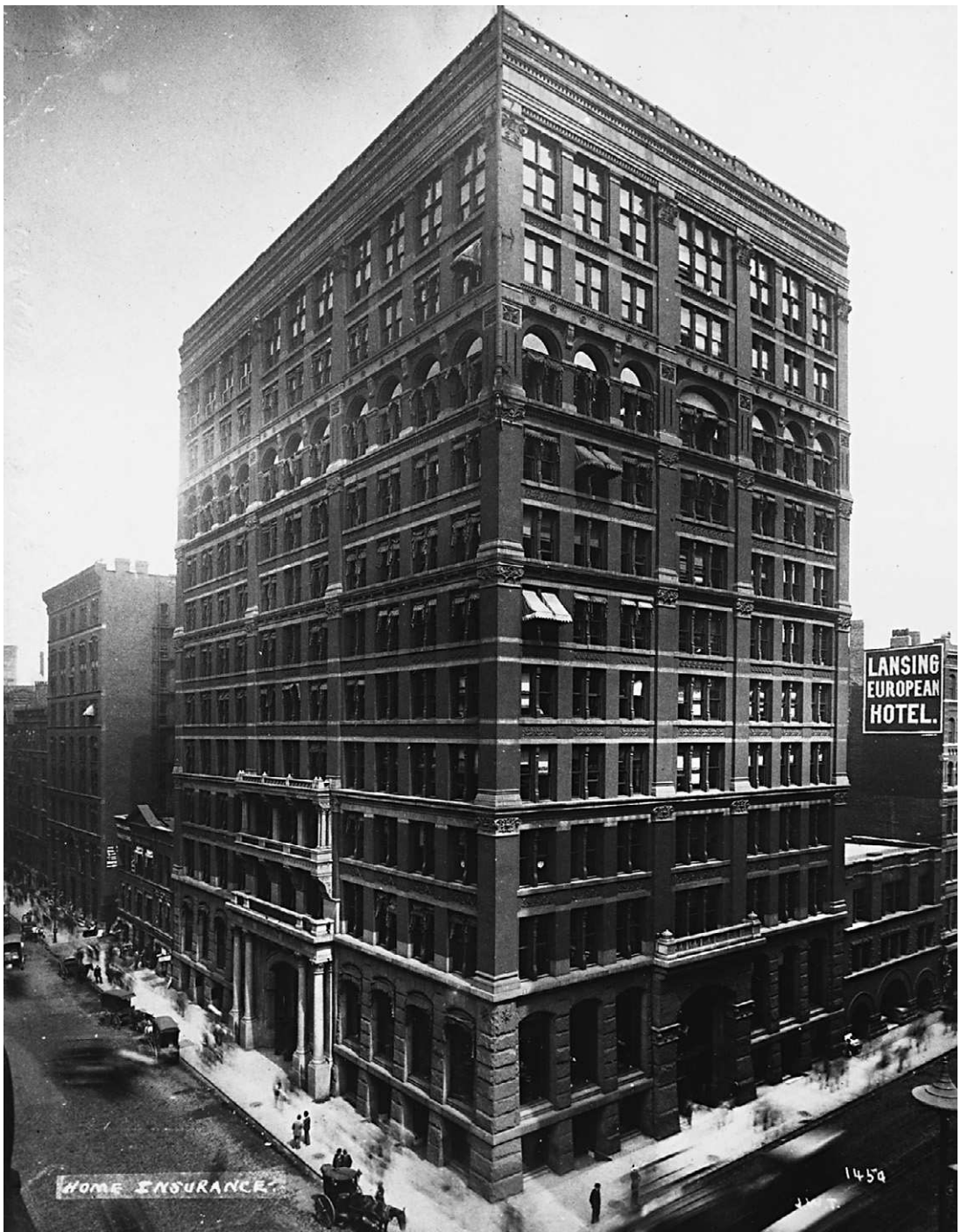
Figure 1.2 Home Insurance Building. This 10-story building, designed by engineer William Le Baron Jenney, is generally considered the world's first skyscraper. Built in Chicago in 1885 using a steel frame, it was demolished in 1931. Courtesy of the Chicago Historical Society.
