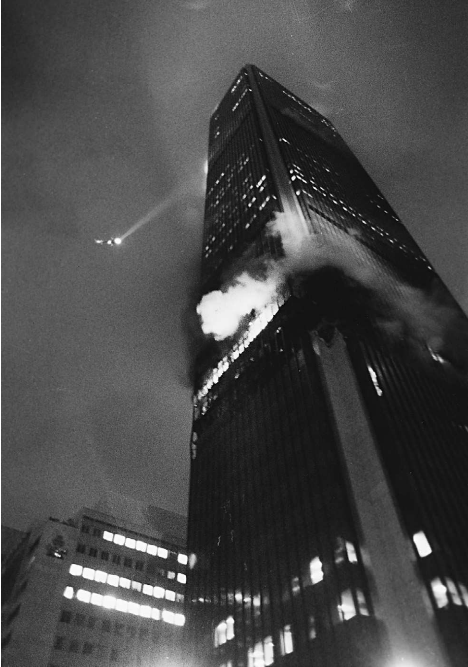
Figure 10.3 TOWERING INFERNO—A fire department helicopter, at left, hovering around First Interstate Bank Building early on Thursday morning, May 4, 1988, as flames shoot from the windows of the 62-story building. Fire officials described the 3½-hour blaze as the worst high-rise fire in the history of Los Angeles. Used with permission from AP/WIDE WORLD PHOTOS.
