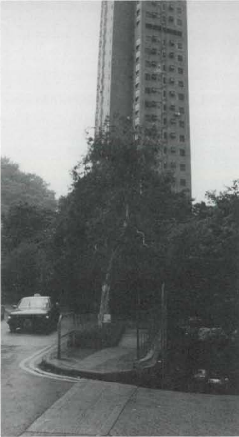
Photograph 4.7 Junction of the access ramp and Kennedy Road which leads to the subject building
