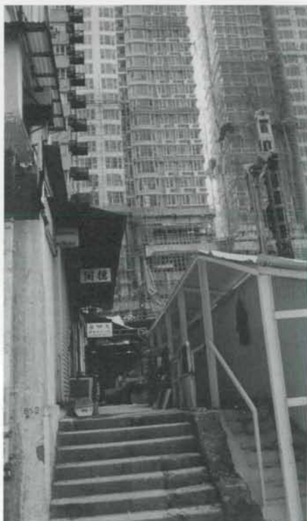
Photograph 4.3 View of Tien Poa Street looking towards Star Street
