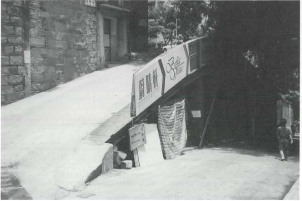
Photograph 4.12 The access ramp off Peel Street leading up to Ying Fai Terrace
