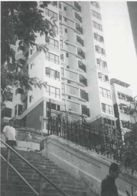
Photograph 4.9 The subject building in the Super Mate (2) Case was completed in September 1999 (view from Ladder Street)
